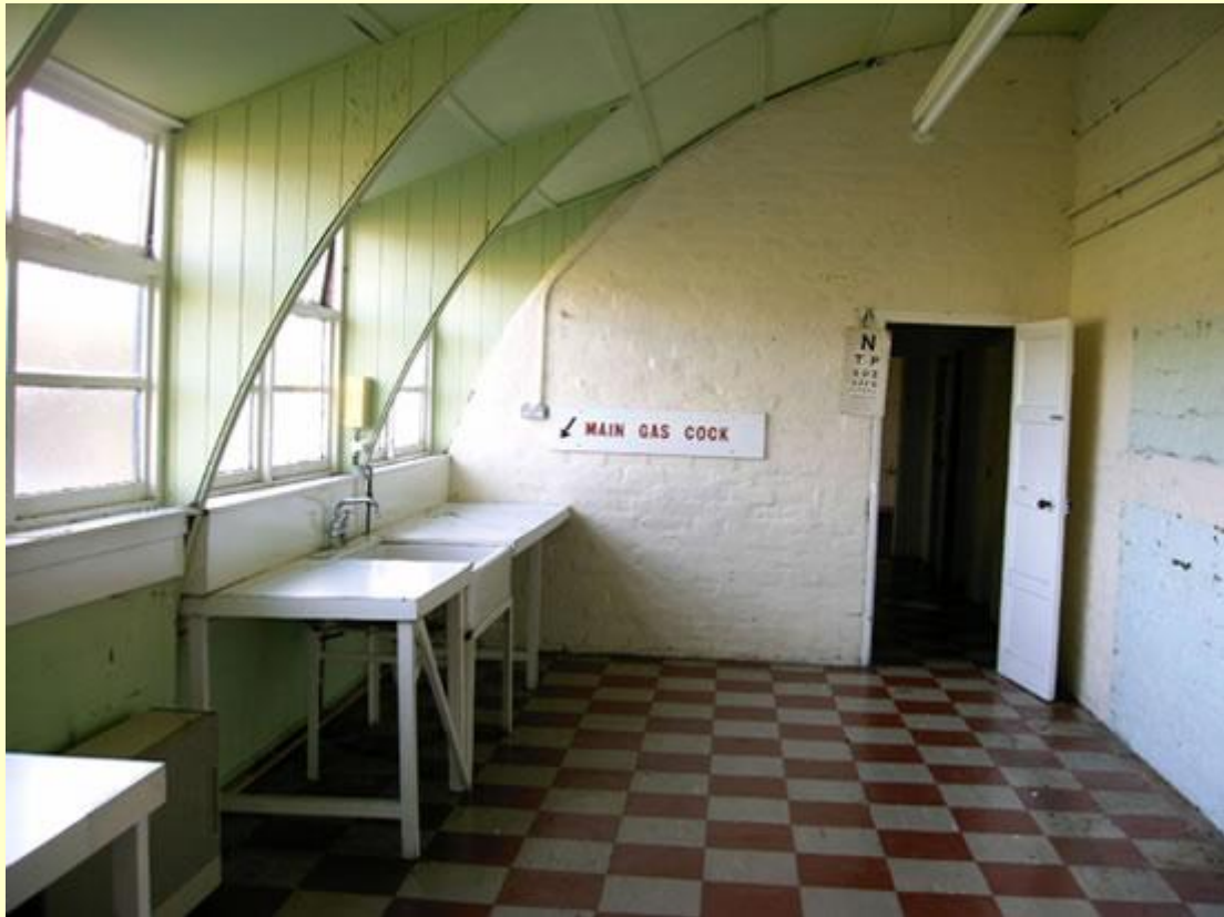
This is the medical centre, built from a 24 foot span Nissen hut and sub-divided internally into many rooms.
