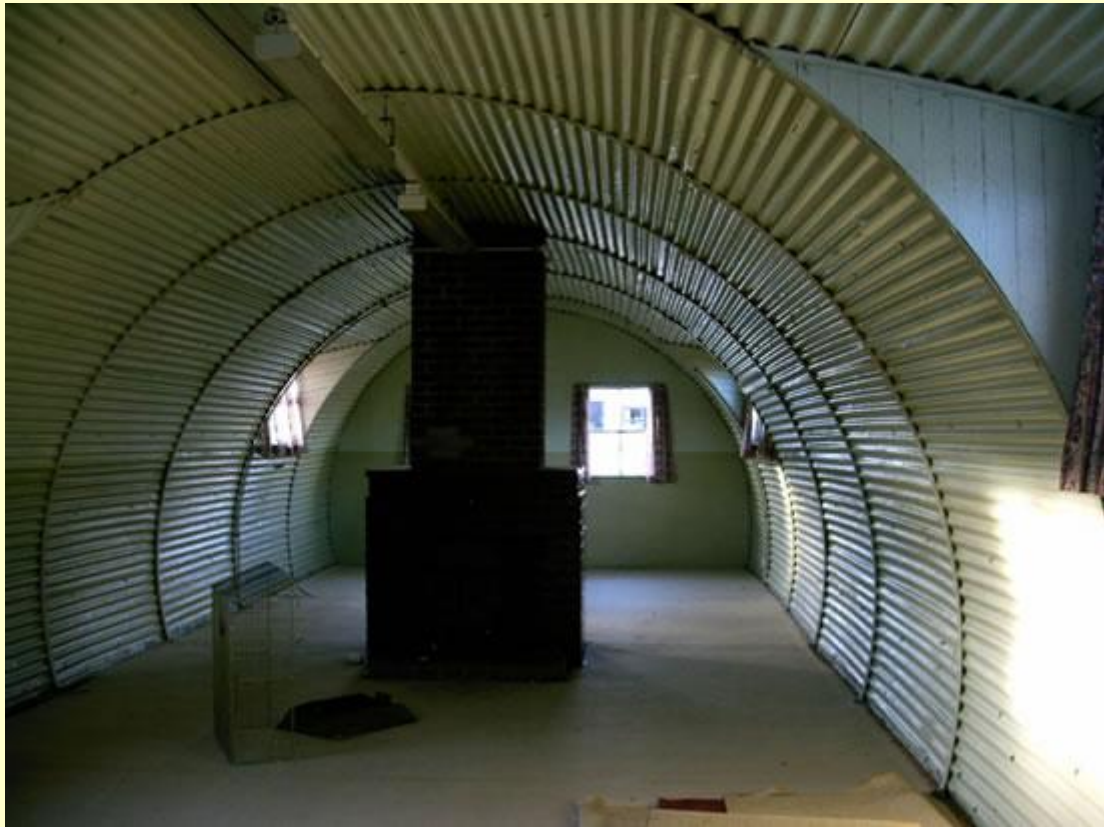
The top shot is of the dining room in the Officer's Mess, while the second one is of the lounge. A bar sits immediately behind the camera in the second photo. Those are original heating stoves in both photos.
